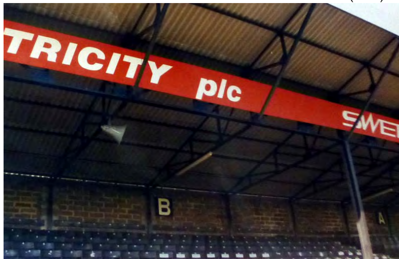
36 1995 CONDITION SURVEY - REC MAIN STRUCTURAL FRAME (BRO) 33
