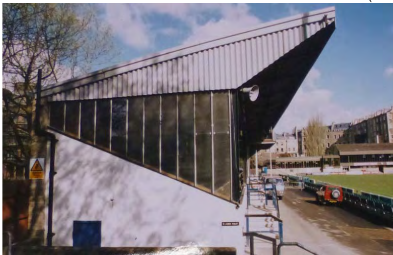
37 1995 CONDITION SURVEY - REC SOUTH ELEV (BRO) 34
