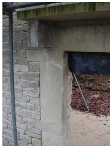
September 2012 – Repaired Door Reveal
