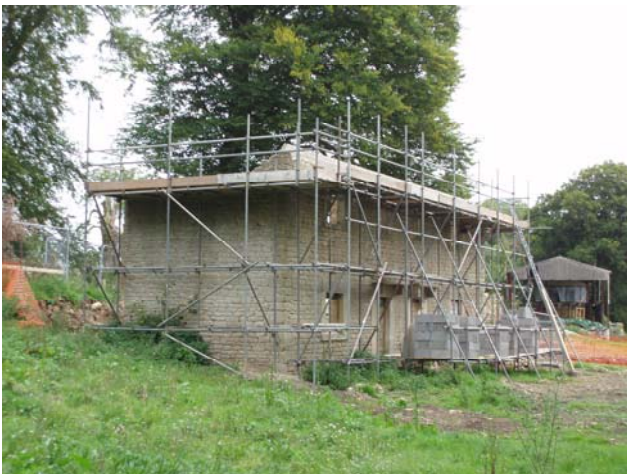
September 2012 – South & West Elevation
