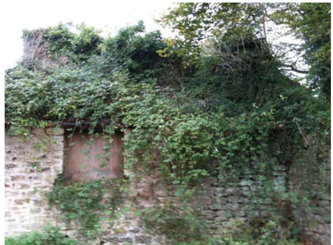
October 2011 – East 'Lean To' Structure
