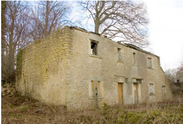
February 2010 - South & West Elevation
