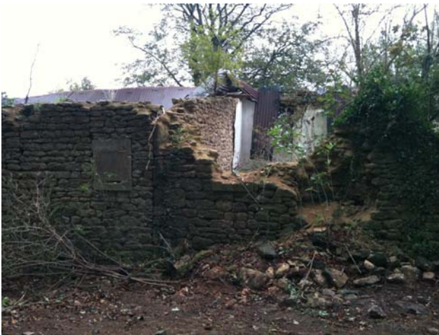
October 2011 - North Elevation
