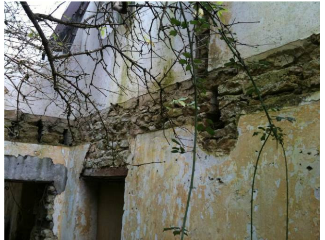
Wall Sockets For Joists/Beams
