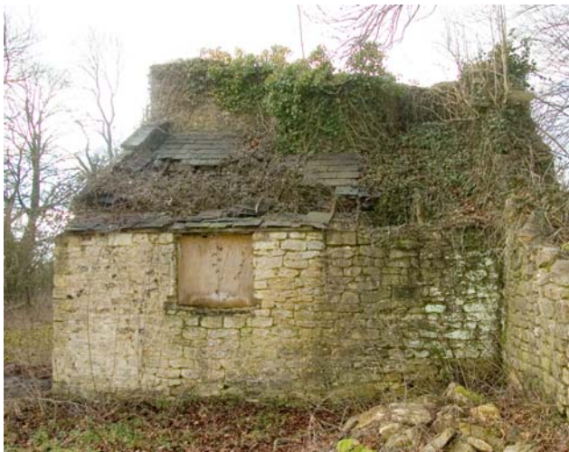
February 2010 – East 'Lean To' Structure
