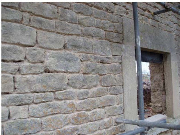
September 2012 - Raked out bed joints
