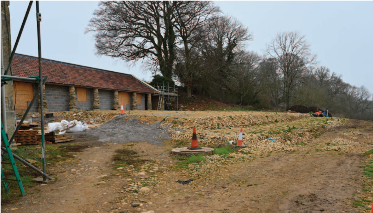
Fig. 14. The restored former open fronted outbuilding at the eastern end of the former farmyard.
