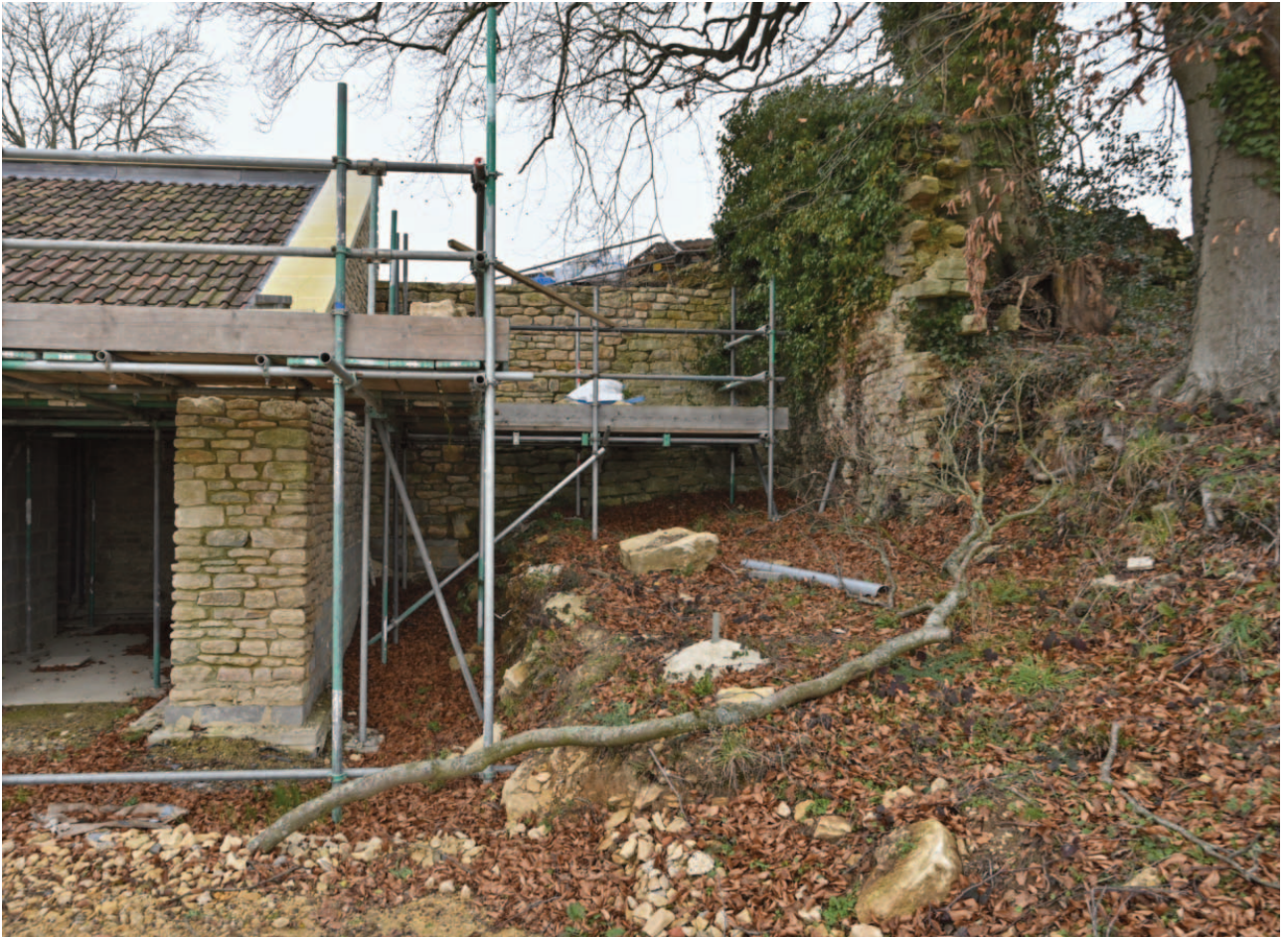
Fig. 21. The end bays of the former open fronted range have not been restored in order to protect the adjacent mature trees whose roots have encroached into the former gable wall.
