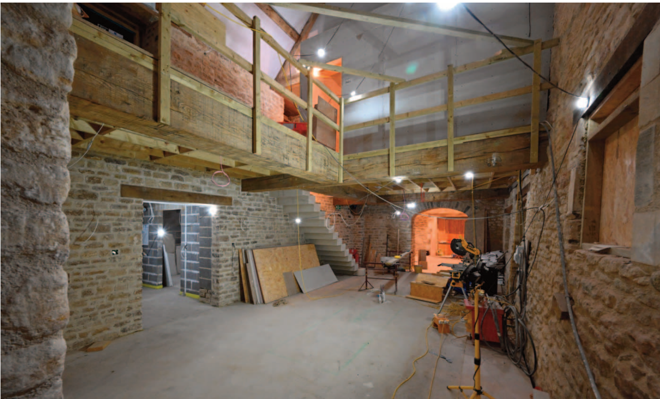
Fig. 25. The approved rebuilt rubblestone faced rear wall within the proposed dining room with the cross barn beyond. The new opening on the left opens into the new below ground extension
