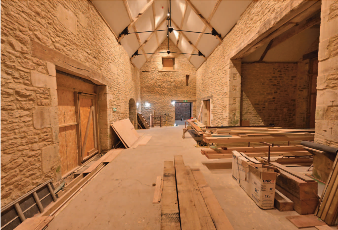
Fig. 26. The full height cross barn without the approved mezzanine and spiral stair at the far end. On the right beyond the midstrey is the new external door opening, and the slightly enlarged opening into the flat roofed rear extension in the far gable.
