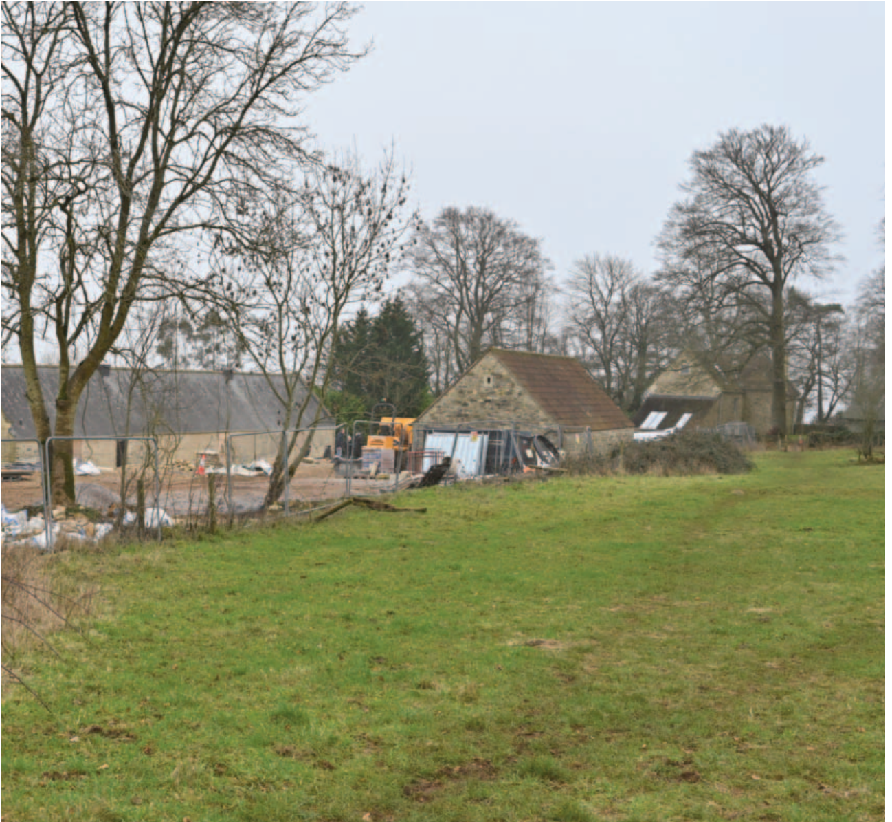
Fig. 10. In contrast to the farmhouse, the former farm cottages on the right are clearly visible from the farmyard and relate closely to it.
