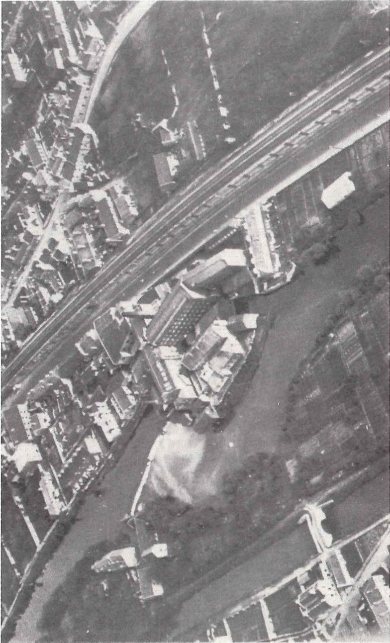
2. Aerial view of Twerton Upper Mill site in 1930. Bamford, Cook & Company's original factory buildings dating from the late eighteenth century form a T-shape in the centre of the complex. (Reproduced by courtesy of the Turner-Messer Twerton Archive)
