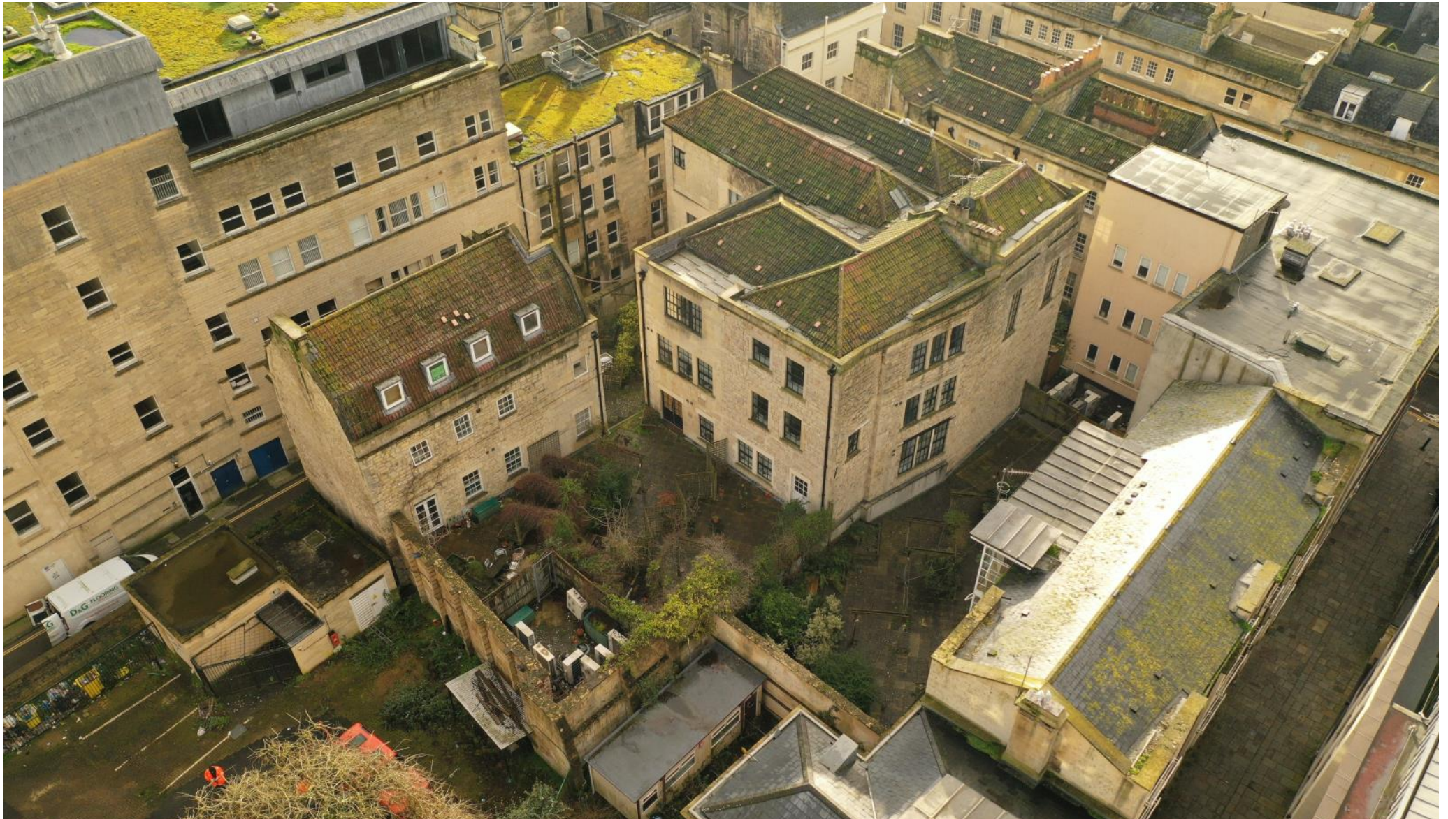
Photo 5: oblique aerial photo showing Nos. 1 and 3 Parsonage Lane in the foreground. The change in levels between the application site and courtyard to Nos. 1 & 3 Parsonage Lane is evident either side of the stone boundary wall.
