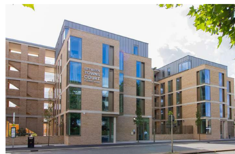
Between Towns Court, Oxford 144 student rooms. Commercial unit, on-site management suite together with associated landscaping and infrastructure. Completed in 2019
