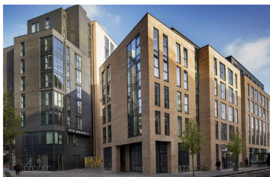
New Bridewell, Bristol 500 student rooms. Ground floor commercial units with associated ancillary facilities and the creation of a new public square. Completed in 2016
