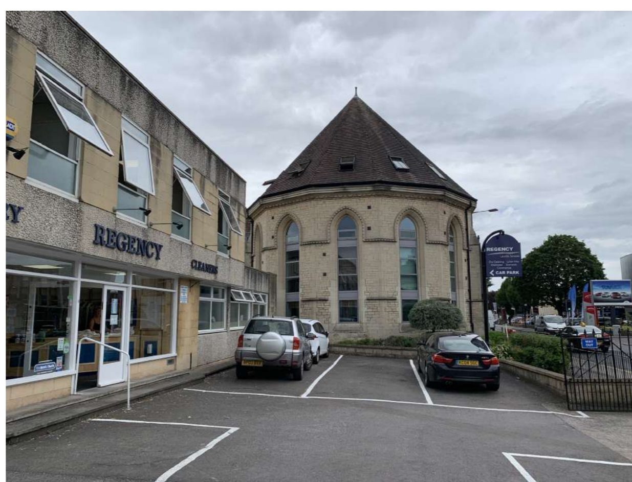
01 View of the Regency Laundry and St Peter's Place from Lower Bristol Road
