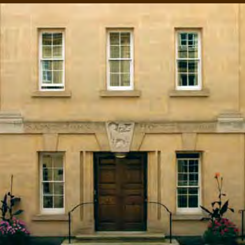
Timber slim-profile double-glazing in the 20th century extension to St John's Hospital
