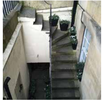
✓ Bath stone steps to basement areas with pennant stone treads and paving.
