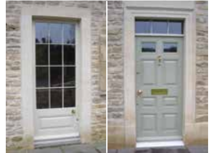
✓ Repaired and refurbished old doors. Images courtesy of Hawker Joinery.
