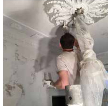
✓ Repairs to plasterwork ceiling rose undertaken by skilled craftspeople.
