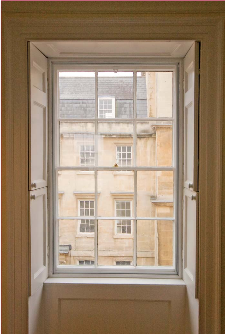
The heat losses through this elegant sash window in the heart of Bath are reduced not only by the shutters (when they are closed) but also by the secondary glazing which sits neatly and discreetly within the window architrave. ©Will Anderson
