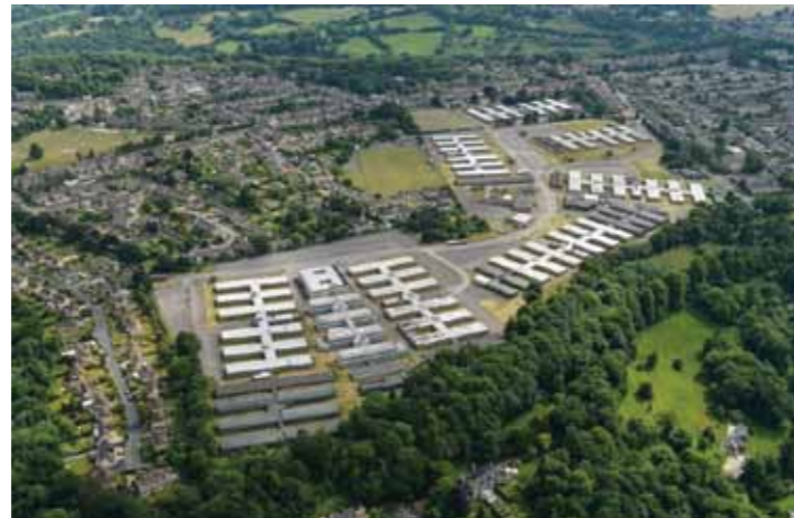
An aerial view of the MOD site looking toward Bradford Road, with Foxhill to the right (Courtesy of Curo).
